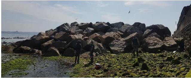
Figure 9: Rock armour breakwater
