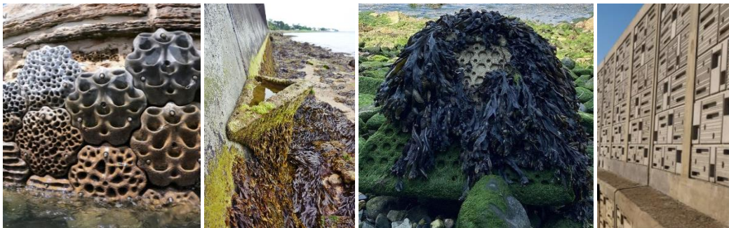
Figure 10: Vertipools, living seawall, eco-blocks and ecoformliners to provide habitat where hard defences are still needed
