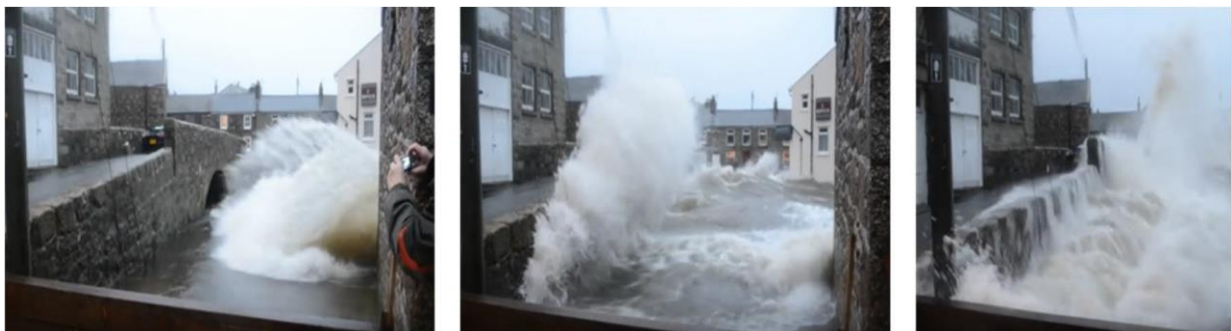
Figure 4: Wave overtopping at Tolcarne bridge, 2014
