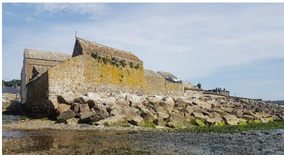
Figure 7: Rock armour revetment in front of wall, Tolcarne Inn
