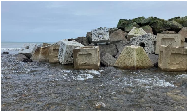
Figure 11: SARCC eco-block NBS pilot
